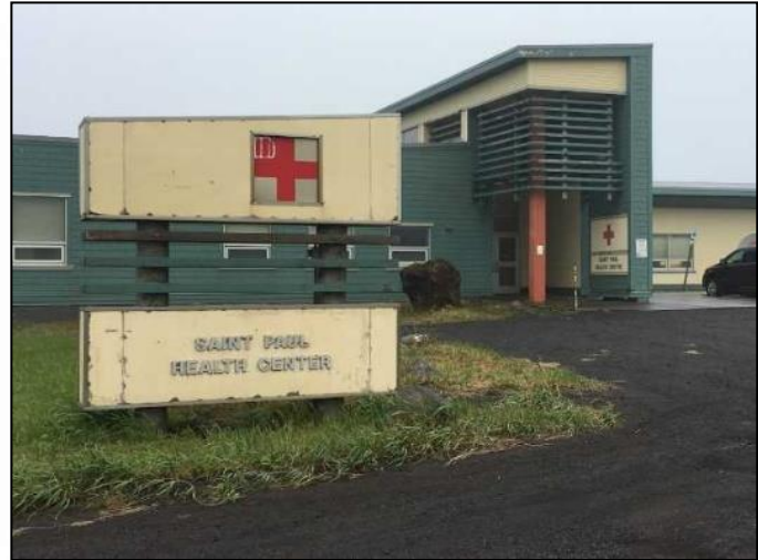
The Saint Paul Community Health Center which is used to provide initial post-crash care in the event of a transportation accident.
