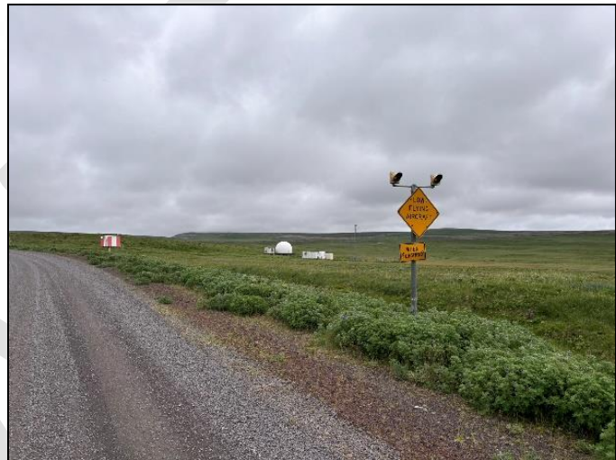
Enhanced roadway safety includes improved traffic control devices that utilize lighting and higher visibility signage.
